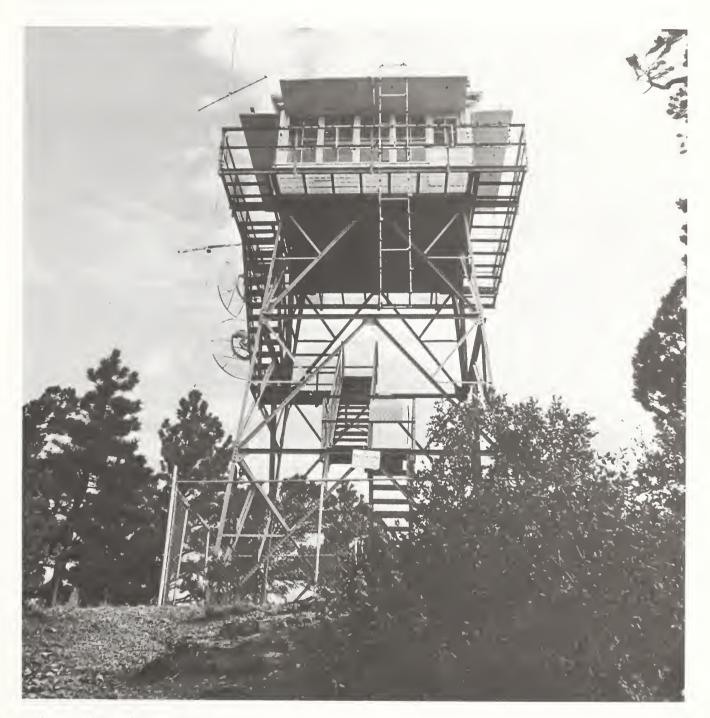
Figure 210. Ruidoso lookout has an Aermotor MI-25, one of only two of that type in the Region.
